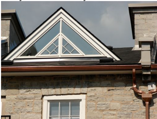
The Prince George Hotel; Triangular Dormers on Clarence Street Façade / Paul Christianson
