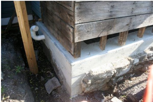
76 Mowat Avenue; raised foundation/ Nicholas Woolley
