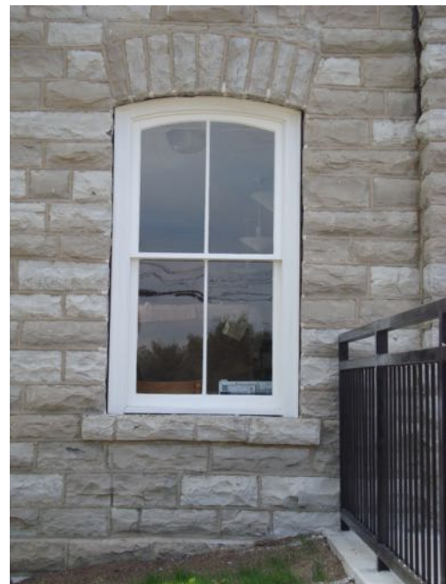
Detail of Window on Entrance Façade / Paul Christianson, 2015
