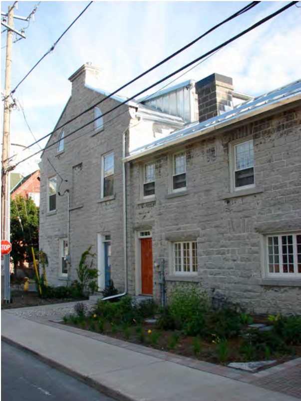
212 King Street East, Earl Street Façade with 44 Earl Street Attached/ Paul Christianson 2009
