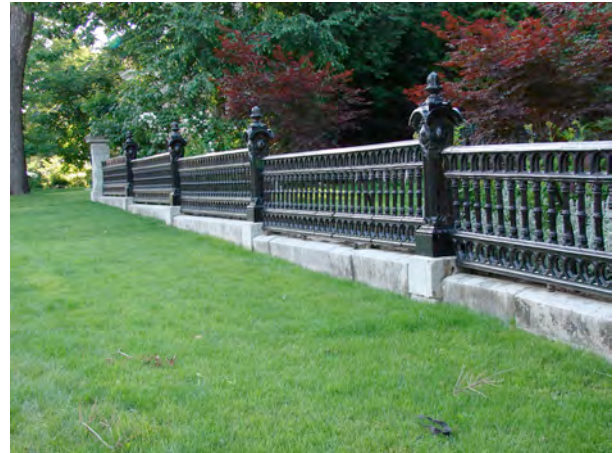
Limestone and Cast Iron Fence at Rosemount/ Paul Christianson 2010
