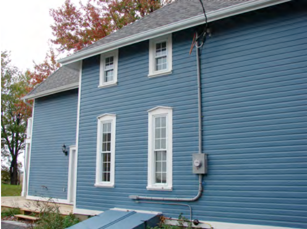
Restored Window Trim, East Façade, Neilson House/ Paul Christianson 2010
