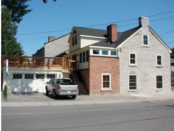
218 King Street East, Earl Street façade/ Paul Christianson 2011
