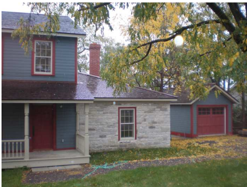
North Stone Addition and Garage
