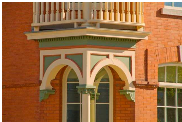
Original and replicated balcony trim..
