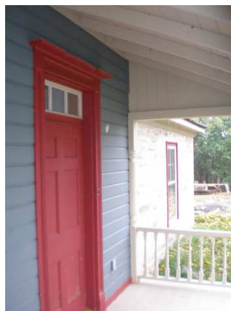
Front Entrance Detail, Photos by R. Crothers
